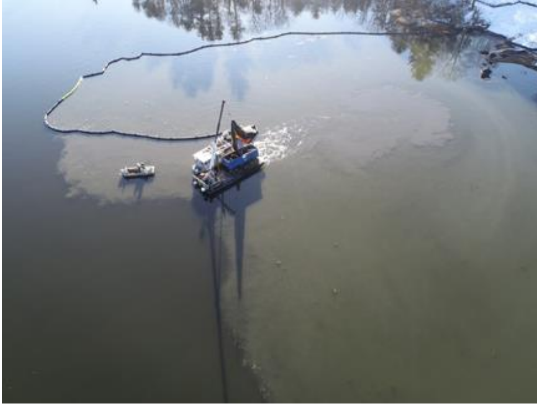
Photo 47. Hand Jet, Flight 6, 12/11/2019. Turbidity barrier removal and dumpster disposal.
