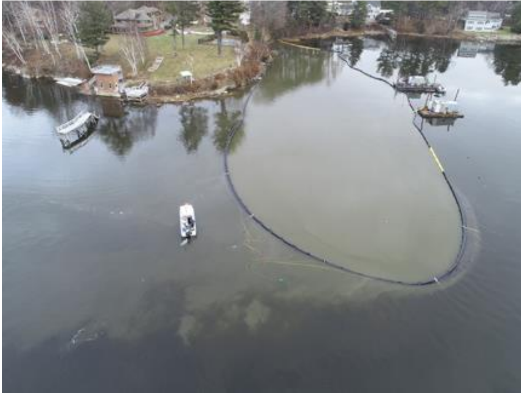
Photo 49. Hand Jet, Flight 8, 12/13/2019. Overfull turbidity barrier on ebb tide on east side. Barrier is briefly spilling at near end. Note water quality sampling boat collecting turbidity profiles in and out of barrier.
