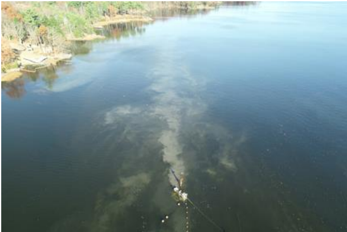
Photo 12. Cable 3, Flight 4, 11/06/2019. Jet plow advancing on western tidal flat, approximately 1 hour after start.
