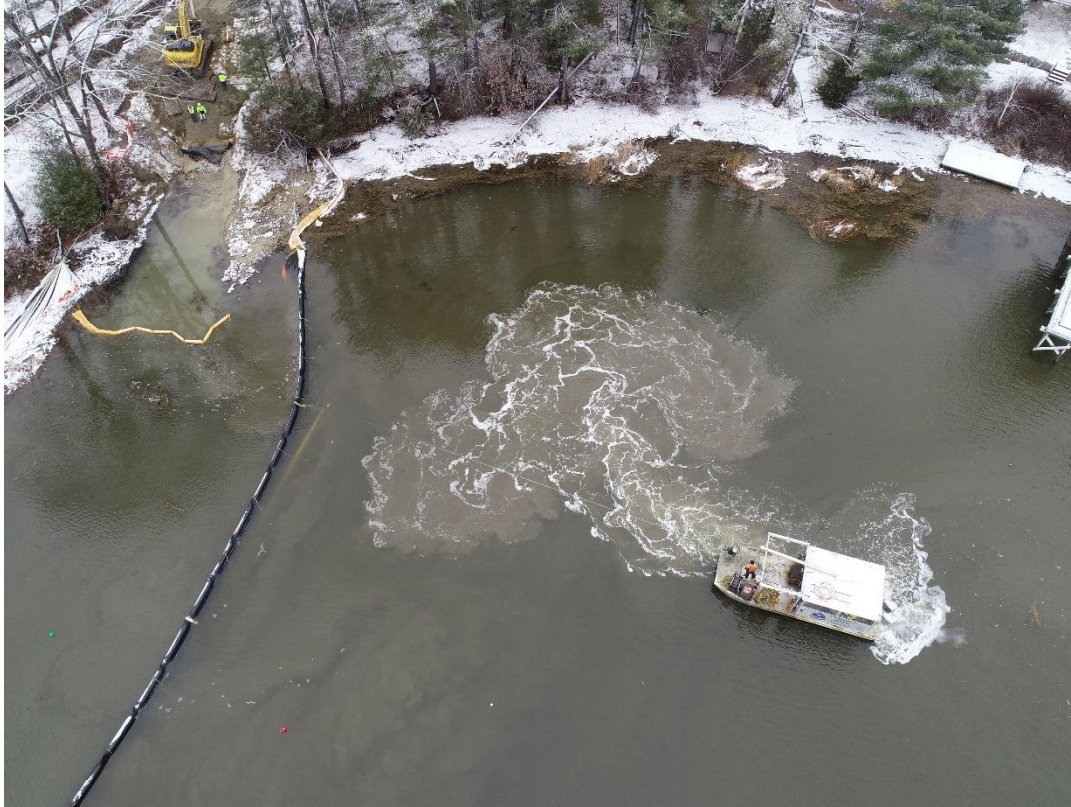
Photo 45. Hand Jet, Flight 1, 12/11/2019. Barge repositioning turbidity barrier.
