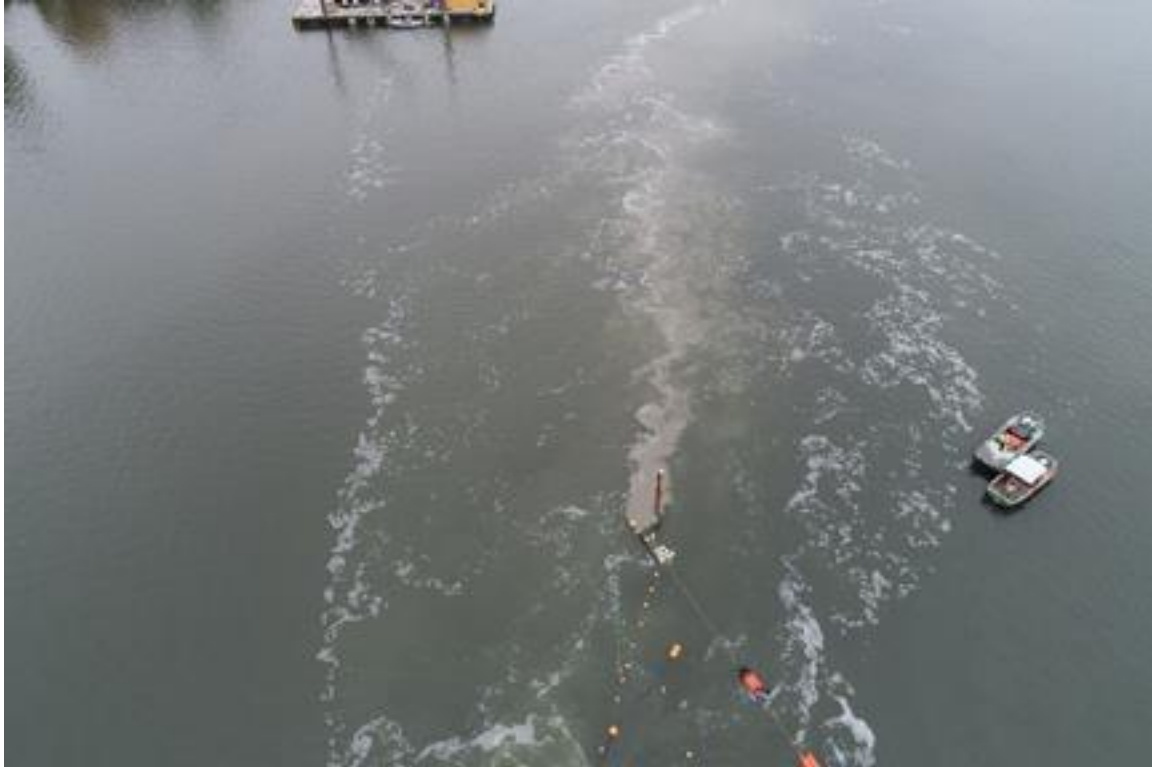
Photo 5. Cable 2, Flight 4, 10/28/2019. Jet burial on western tidal flats. Note narrow linear turbidity plume.
