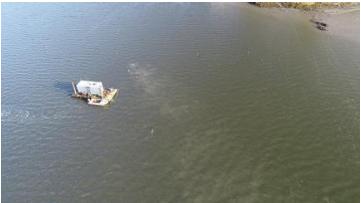
Photo 38. Hand Jet, Flight 1, 11/15/2019. Diver burial on channel slope on east side. Note diver air bubbles at top of sediment plume.
