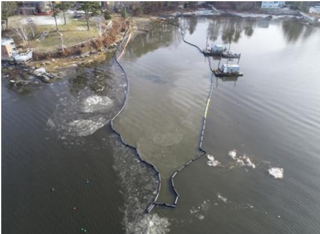
Photo 48. Hand Jet, Flight 2, 12/13/2019. Skim ice piling up against turbidity barrier on flood tide.
