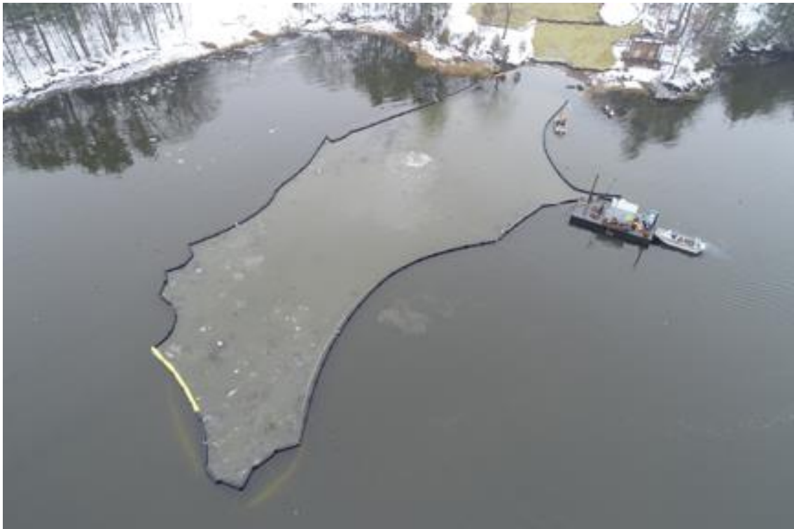
Photo 44. Hand Jet, Flight 2, 12/09/2019. Diver burial in west side turbidity barrier on a flood tide, showing icy conditions.
