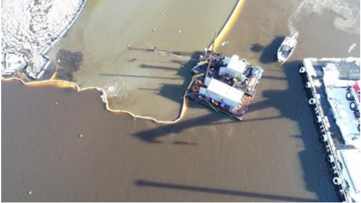
Photo 55. Hand Jet, Flight 2, 12/18/2019. Type 1 curtain on flood tide. Note turbid water in bay from storm event.
