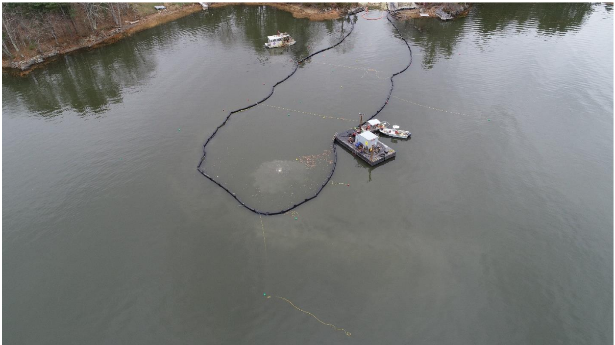
Photo 34. Hand Jet, Flight 1, 11/14/2019. Western tidal flats, diver working inside turbidity barrier on an ebb tide.
