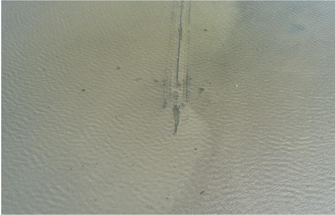
Photo 3. Jet Plow Trial, 9/9/2019. Jet plow track showing start of jet plow. For scale, the combined width of the two skids are approximately 15 ft wide.
