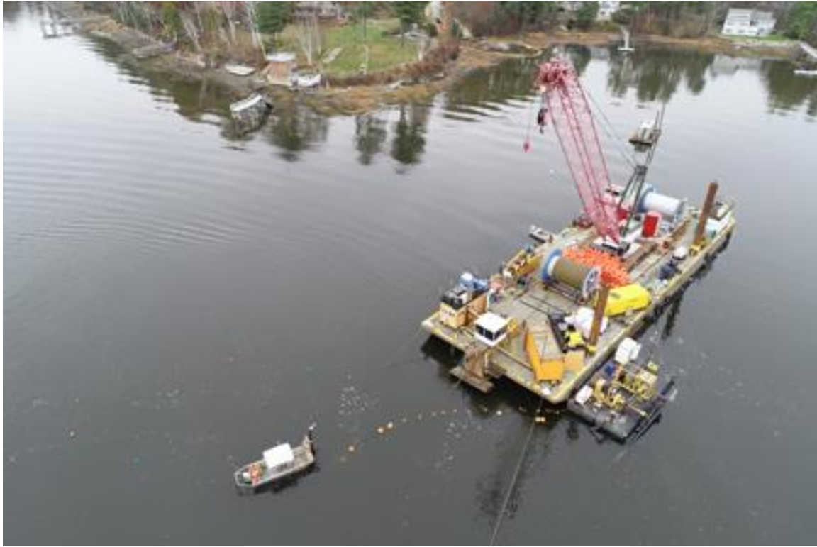
Photo 29. Cable 3, Flight 12, 11/07/2019. Completing jet plowing on east side.
