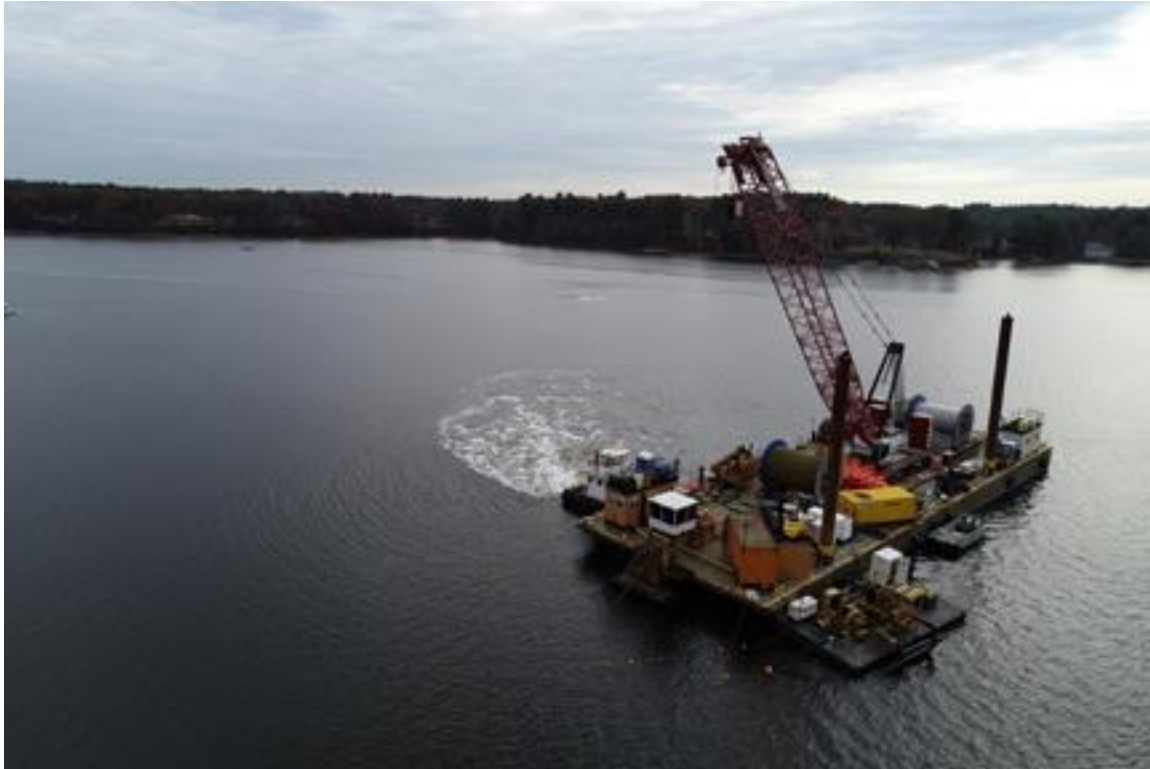
Photo 23. Cable 3, Flight 3, 11/07/2019. Jet plow burial in channel; no visible plume.
